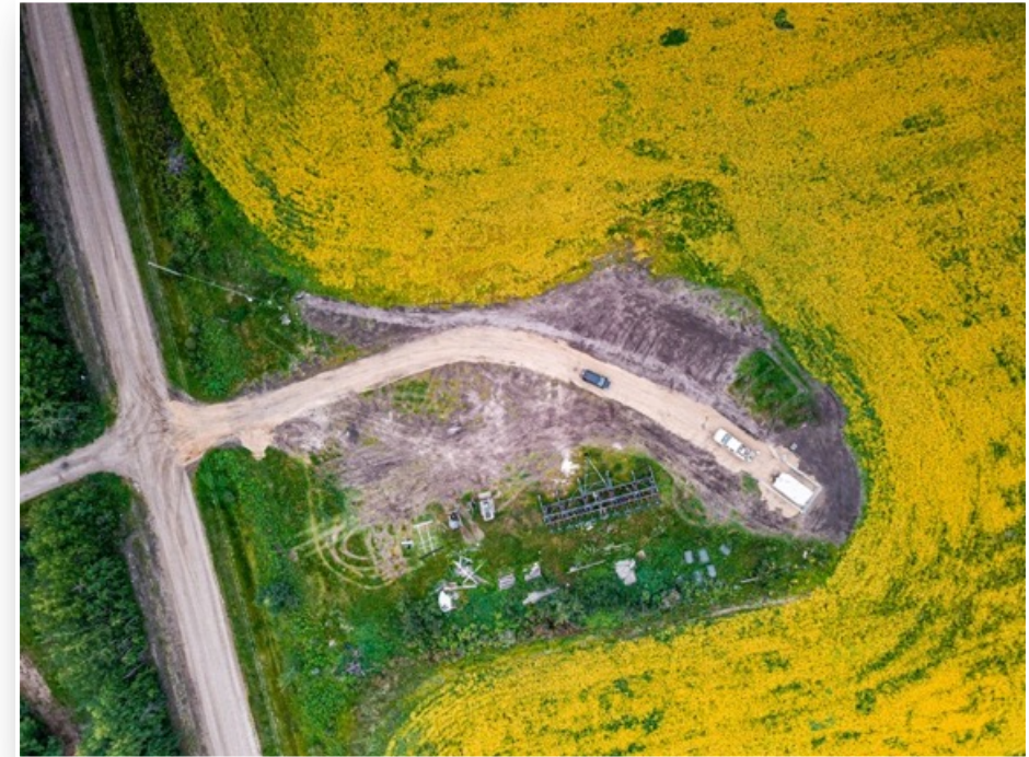
Overhead view of Station 986c deployment
