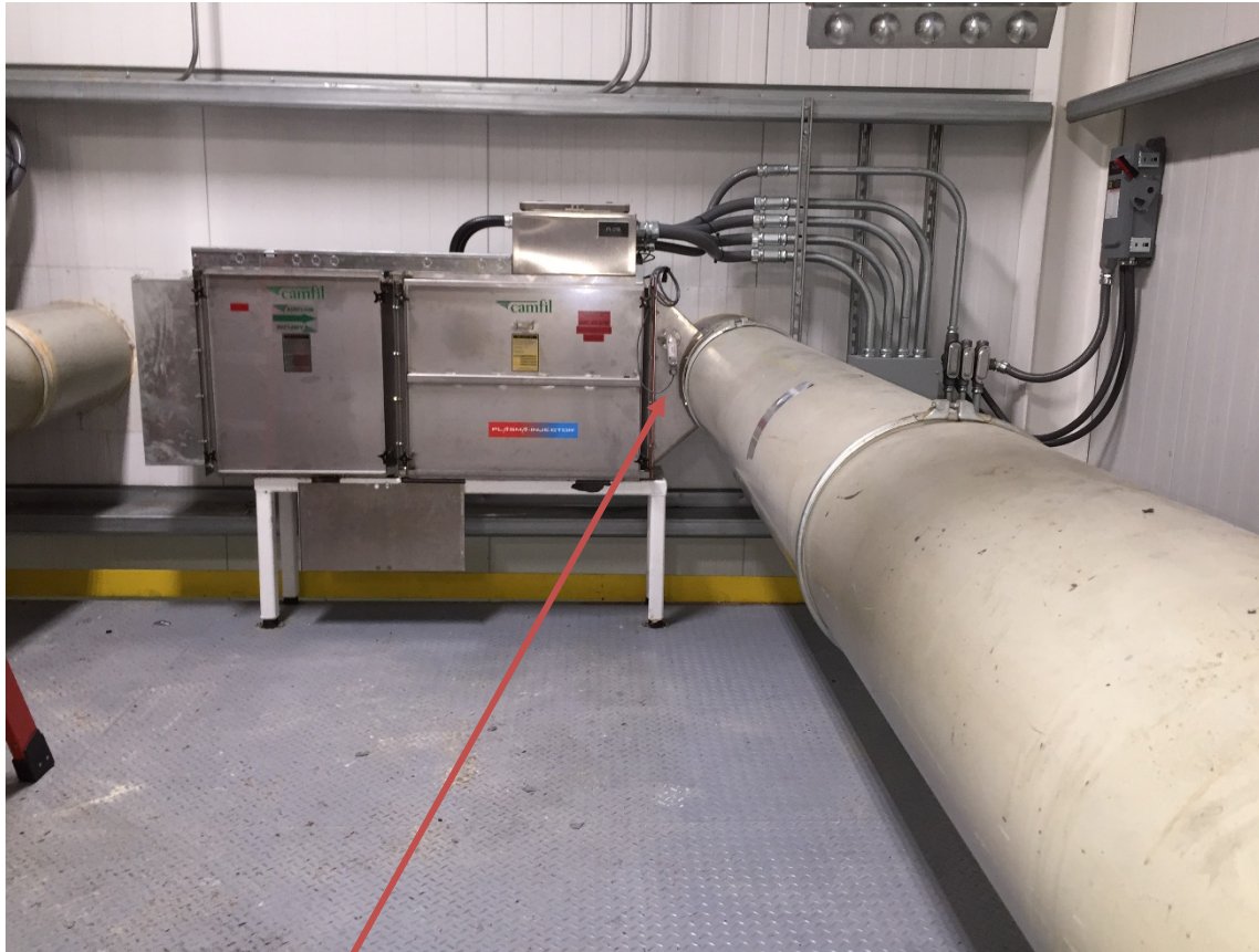
T'-adapter connecting Plasma-Injector to exhaust duct
